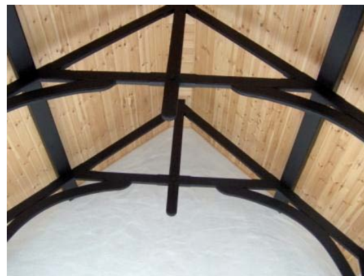
Vaulted roof in conservatory
